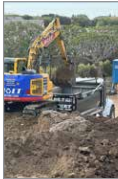
Excess dirt will be used for new lawn area.
