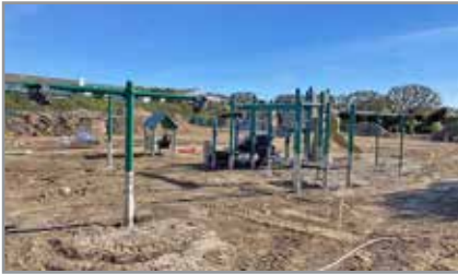
Playground area ready for expansion and rubber surface.
