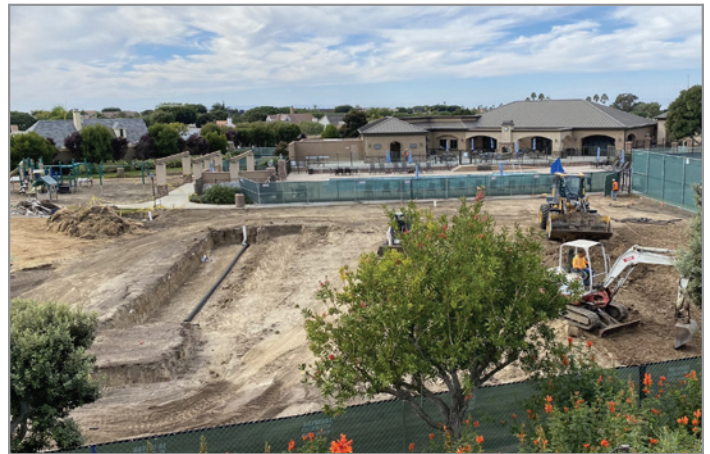
Amenities work continues in the Community Center Park.
