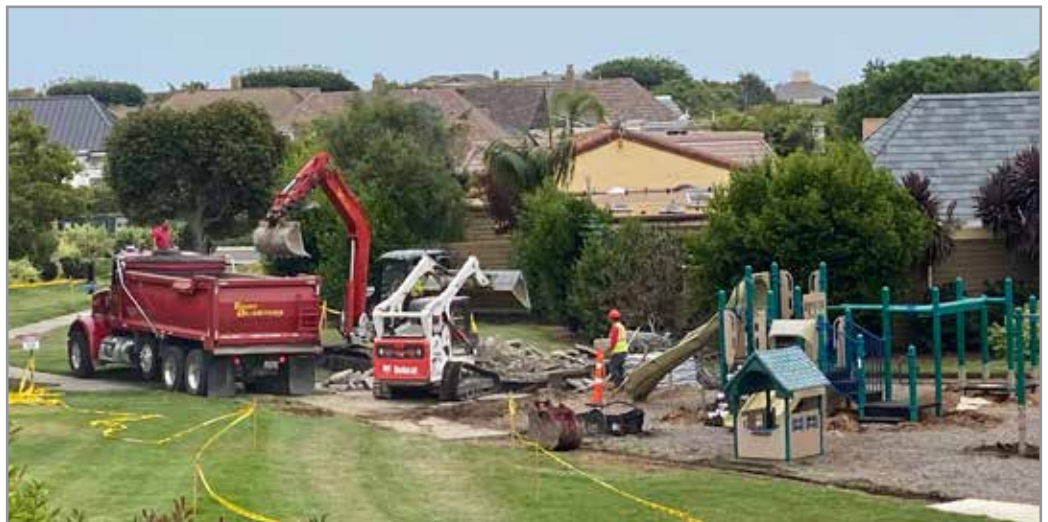
Playground improvements in progress.
