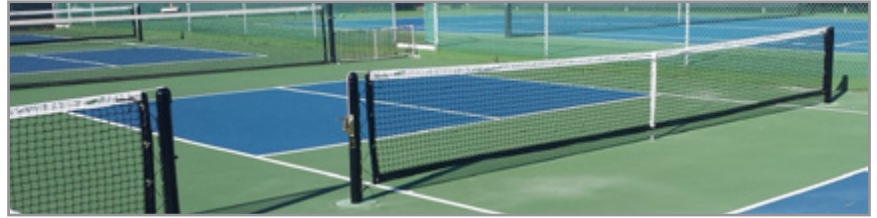
Installation of new Pickleball nets. Photos by Don Baer
