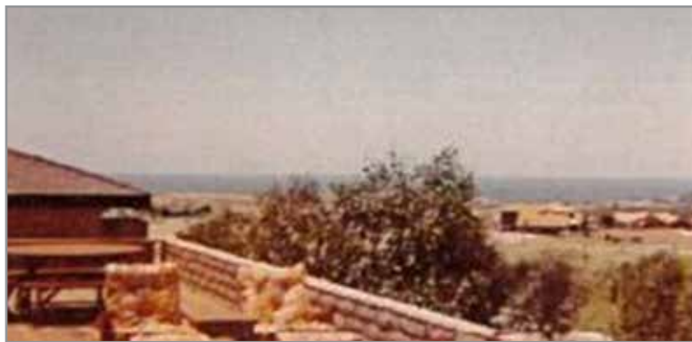
View of bare hills and construction trailers from Brigantine Drive.
