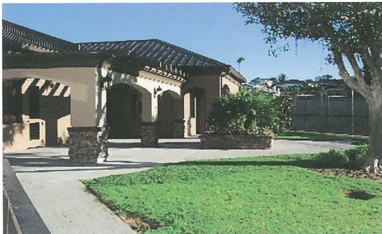
Rear view of the new Niguel Shores office
