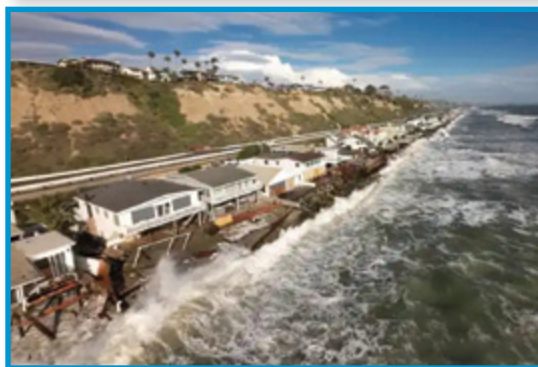
High surf damaging Dana Point homes, September 8.
