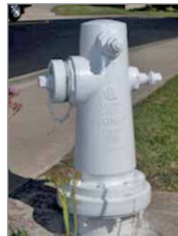
Newly painted NSCA fire hydrant.
