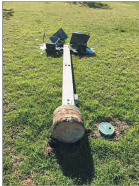
Wind damaged Coach Light
