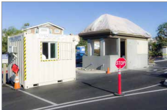
Gatehouse Renovation with Temporary Entrance Facility
