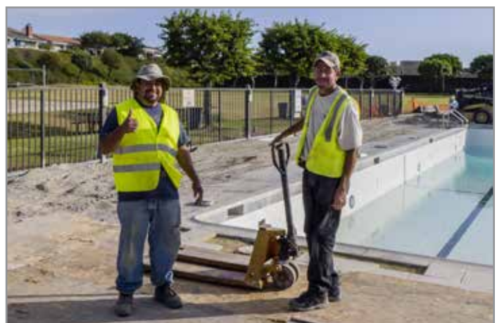
Pool deck renovation with pool deck renovators.
