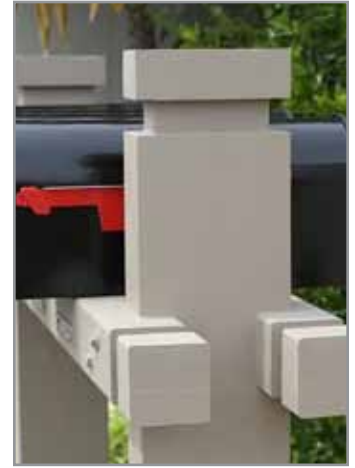
Repaired Mailbox Post
