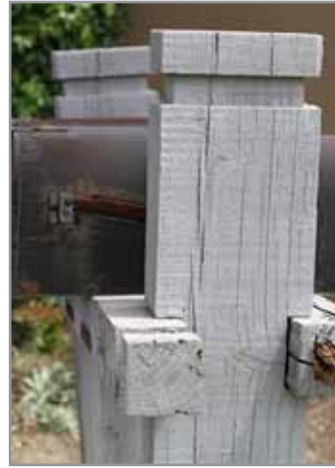
Deteriorated Mailbox Post
